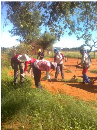
Top Village before clearing
