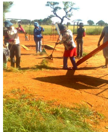
During the Clearing at Top Village
