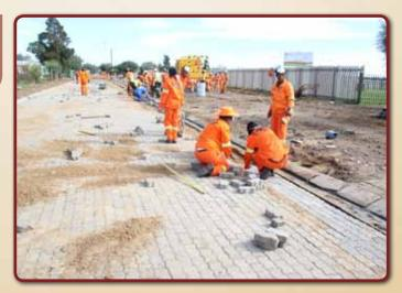
which is one of the gravel streets in the area. The activities taking place on the site include road earth works, pavement layerworks, road surfacing (concrete segmented paving blocks) and the provision of storm water infrastructure.
